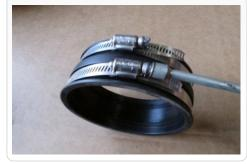
19. Slide the coupler with both hose clamps onto and over the intake tube. Push the coupler past both stop beads leaving the end of the tube exposed.
