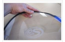
**44.** Once edge trim is installed roll the sides of the lid on a flat surface to ensure a tight seal.
